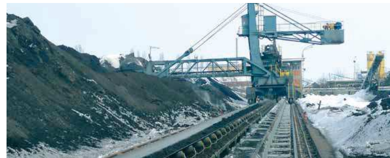
Extremely dirty and tough environment in coal handling. igus® roller e-chains® guided in tough steel troughs
